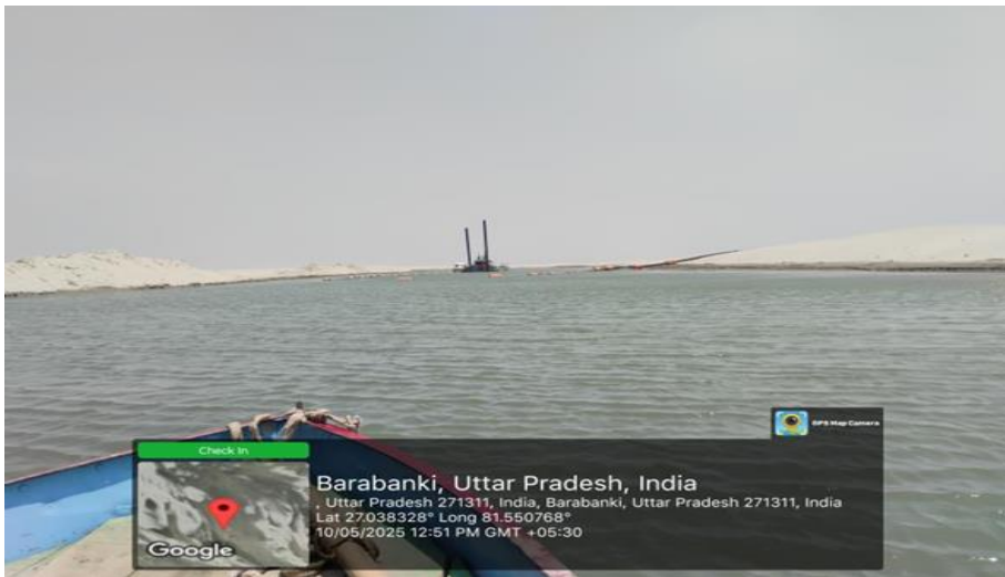
Fig. 1(a). Dredged channel at Ghaghara River, Barabanki District (Siroli Goong Village site)
