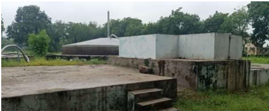
Figure: 1 Bio-Gas Plant
